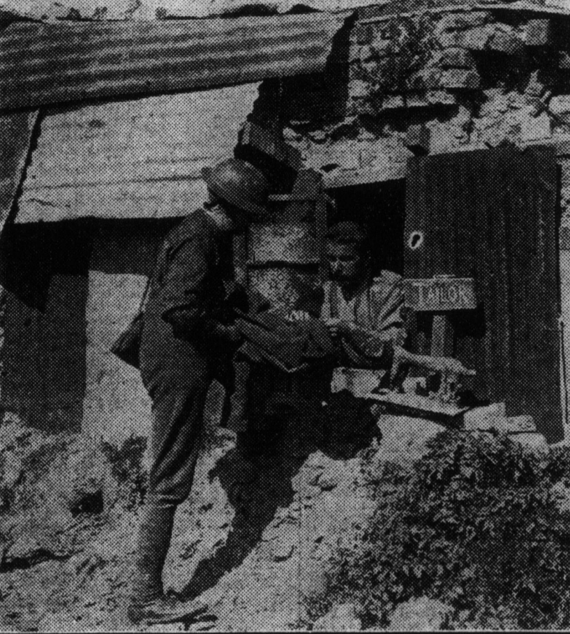
This Canadian official photograph shows a Canadian, about to go on leave, taking his tunic to the tailor's shop for alterations. The shop is made of salvaged iron, boards and bricks. The sign is an old sewing machine found among the ruins of a village.
