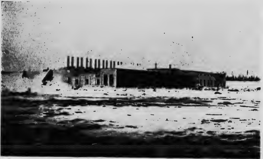
Winnipeg Electric Railway Company, Power House on Pinawa Channel, Winnipeg River.
