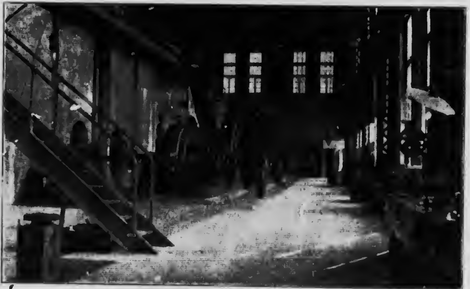
Kenora Power Station, Interior.
