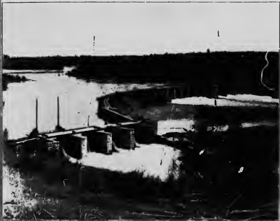
Winnipeg River, Norman Dam Controlling Outlet Lake of the Woods.
