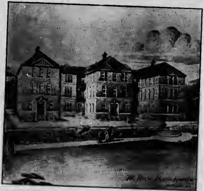
NEW HOSPITAL, formally opened by H.R.H. Duke of Connaught, September 17, 1912
