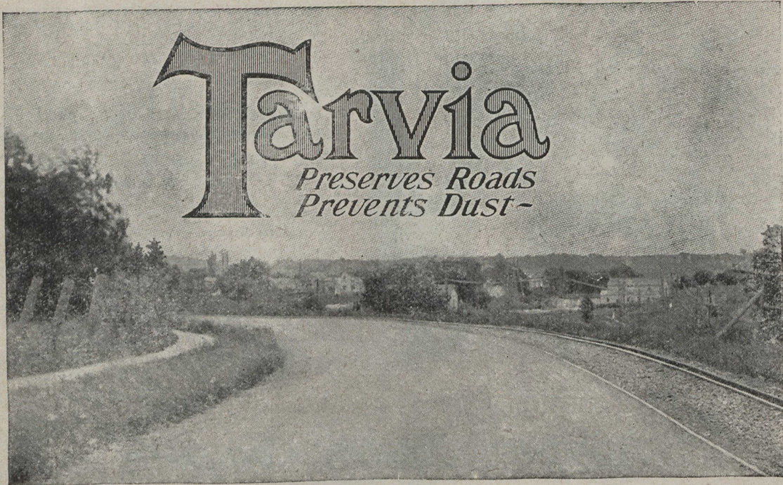
Merrilton Road, St. Catharines, Ont. Resurfaced with "Tarvia-X" and with "Tarvia-B" seal coat in 1917.
