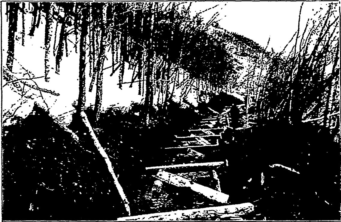
Constructing Flume on McKee Creek for the Atlin Mining Company, Atlin, B.C.
