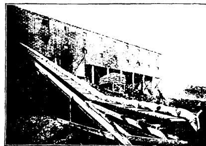
Freight and Package Elevator
