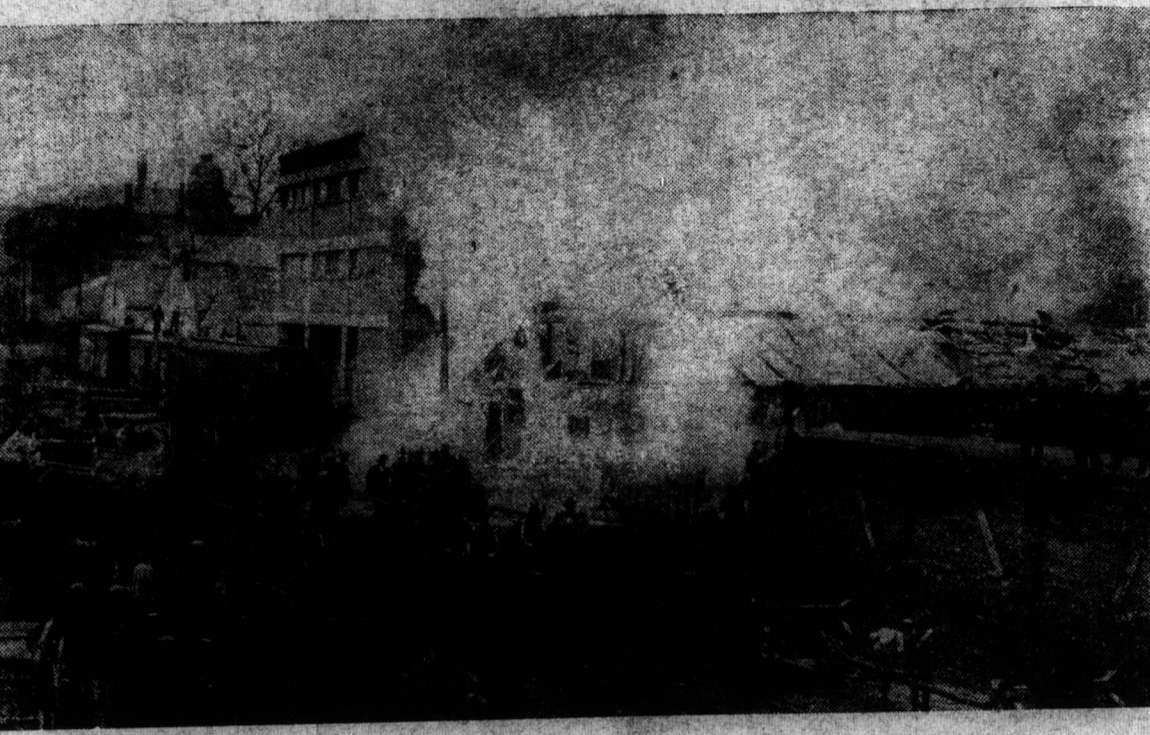
The above is the scene of last night's fire on Colborne street, when the Anguish livery barn was destroyed by fire. The building was one of the city's landmarks, and will be replaced by a modern structure.
