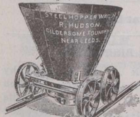
27—Hopper Wagon, with Slide Door
