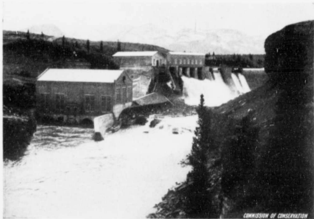
CALGARY POWER CO.—HORSESHOE FALL HYDRO-ELECTRIC PLANT, 50 MILES WEST OF CALGARY, ALTA.
