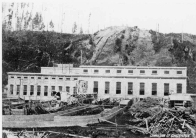
BRITISH COLUMBIA ELECTRIC RAILWAY CO.—JORDAN RIVER HYDRO-ELECTRIC PLANT, 43 MILES WEST OF VICTORIA, B.C.
