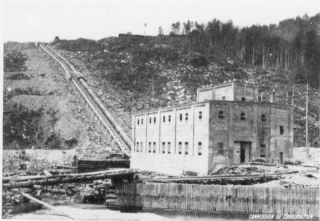
NORTHERN ONTARIO LIGHT AND POWER CO.—HYDRO-ELECTRIC PLANT, MATABITCHUAN RIVER, TIMISKAMING DIST., ONT., 25 MILES SOUTH OF COBALT, ONT.
