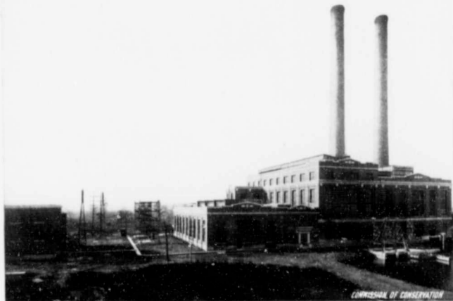
DOMINION POWER AND TRANSMISSION CO., AUXILIARY STEAM PLANT, HAMILTON, ONT. Largest auxiliary plant in Canada. 20,000 k.w. in steam turbine units.
