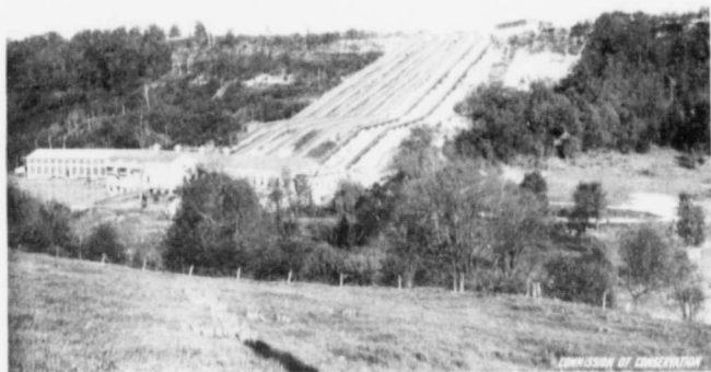
DOMINION POWER AND TRANSMISSION CO.—HYDRO-ELECTRIC PLANT AT POWER GLEN, 33 MILES EAST OF HAMILTON, ONT.
