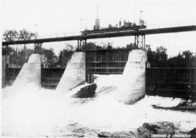
CONTROL SLUICE GATES, SHAWINIGAN WATER AND POWER CO., SHAWINIGAN FALLS, RIVER ST. MAURICE, ST. MAURICE CO., QUE.
