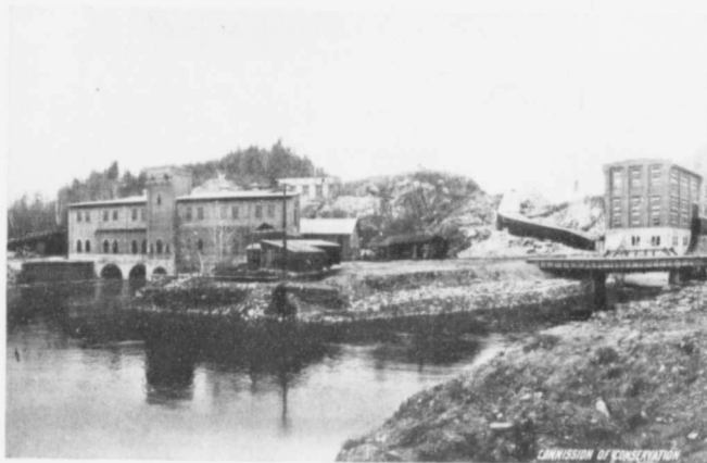
CANADIAN COPPER CO.—TWO HYDRO-ELECTRIC PLANTS ON SPANISH RIVER, 30 MILES SOUTHWEST OF COPPER CLIFF, SUDBURY DISTRICT, ONT.
