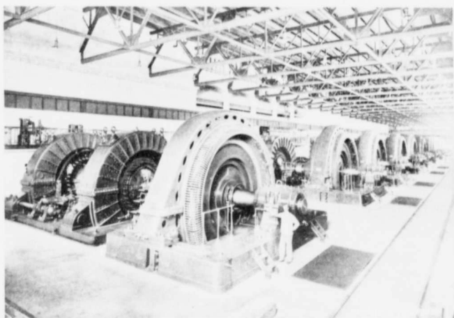
ONTARIO HYDRO-ELECTRIC POWER COMMISSION.—HYDRO-ELECTRIC PLANT AT NIAGARA FALLS, ONT.
