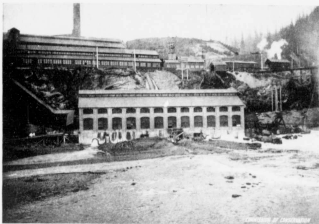
GRANBY CONSOLIDATED MINING, SMELTING AND POWER CO.—HYDRO-ELECTRIC PLANT AT ANYOX, OBSERVATORY INLET, B.C.
