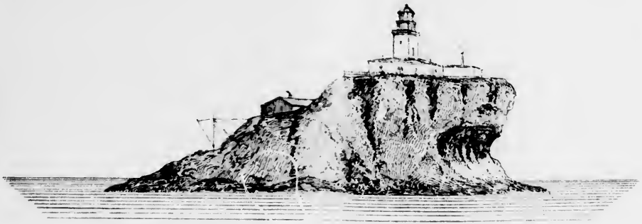
Tillamook Rock Light-house (as seen from the northwestward). Fog-siren.
