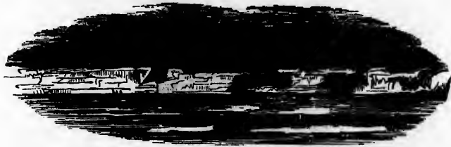
EXCESSIVE REFRACTION OF BERGS.
