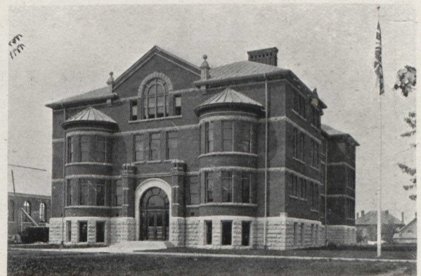
Peterborough High School, Peterborough. Mr. Belcher, Architect. Mr. Duranceau, Plumber.
