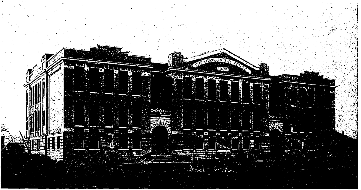
The George Jay School, Now Being Built by the Board of Education at Victoria, B.C. In the Plan and Construction of This Building the Essentials of School Hygiene and the Safety of the Scholars Have Been Thoroughly Considered. The Exterior Walls are of Concrete and Pressed Brick, the Interior Dividing Walls and Partitions of Brick and Hollow Tile; and the Beams, Floors, Roof and Stairs of Reinforced Concrete. Thos. Hooper, Architect.
