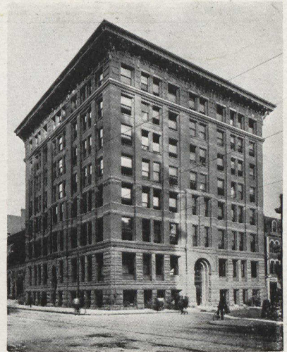
Continental Life Building, Bay Street, Toronto. Mr. Tellier, Architect. Purdy-Mansell, Plumbers.
