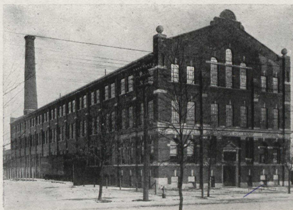
Sunbeam Incandescent Lamp Co.'s Building, Dufferin Street, Toronto. F. Herbert, Architect. W. J. McGuire, Limited, Plumbers.
