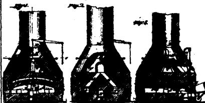
5314 Stevens & Cross' Furnace for making Wrought Iron direct from the Ore.
