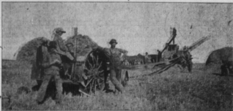
"Waterloo Boy" Tractor operating Threshing Outfit on the Farm of W. J. Duke, Dollard, Sask.
