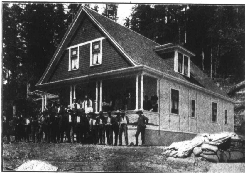
Queen's Hospital, Rock Bay, B.C.
