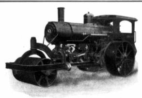
SHOWING AVERY DOUBLE UNDERMOUNTED TRACTION ENGINE FITTED AS A ROAD ROLLER.
