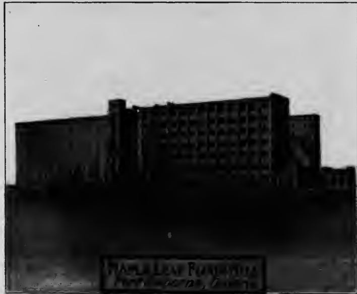
Two of the eight mills of the Maple Leaf Milling Company, having a total capacity of over 15,000 barrels daily.
