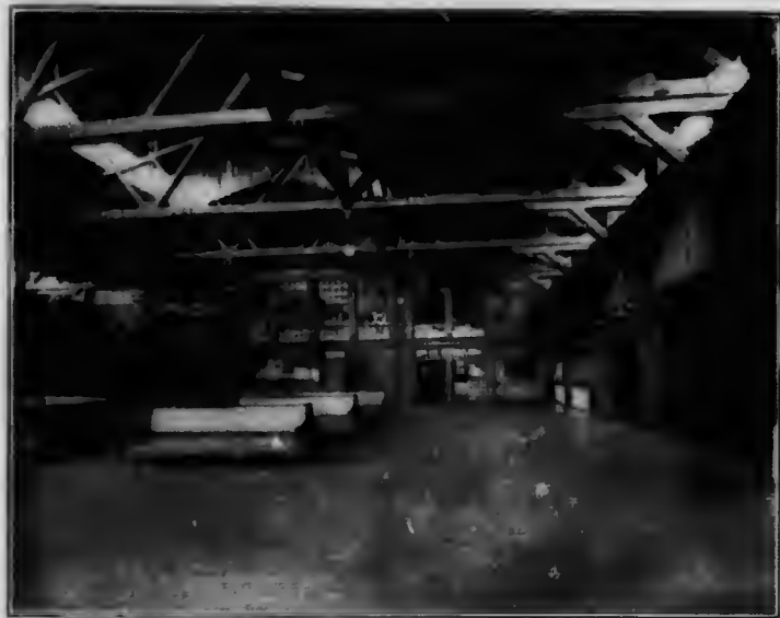
Example of Douglas Fir as structural material in reception room, C.P.R. dock, Vancouver.
