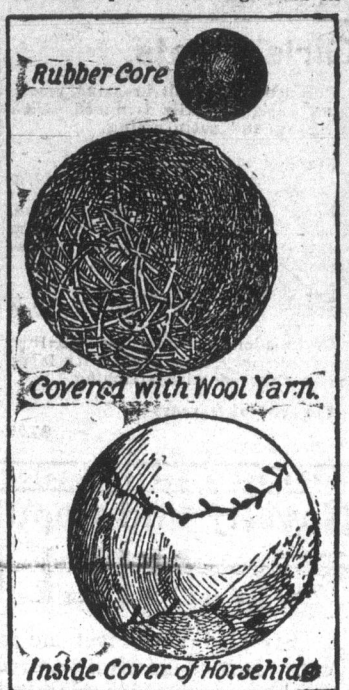
THE EARLY STAGES OF A BASEBALL DURING MANUFACTURE.
