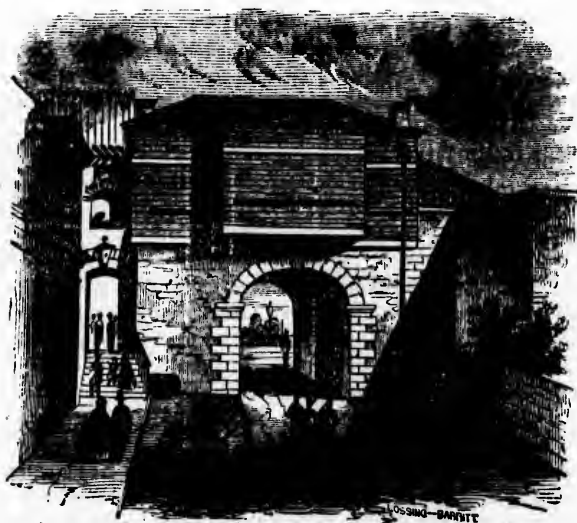
PRESCOTT GATE, DEMOLISHED, AUGUST, 1871.
