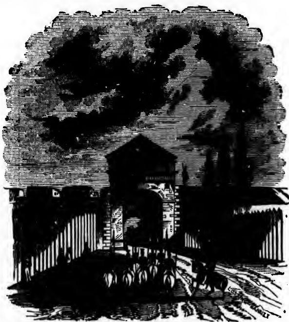
ST. LOUIS GATE, DEMOLISHED, AUGUST, 1871.
