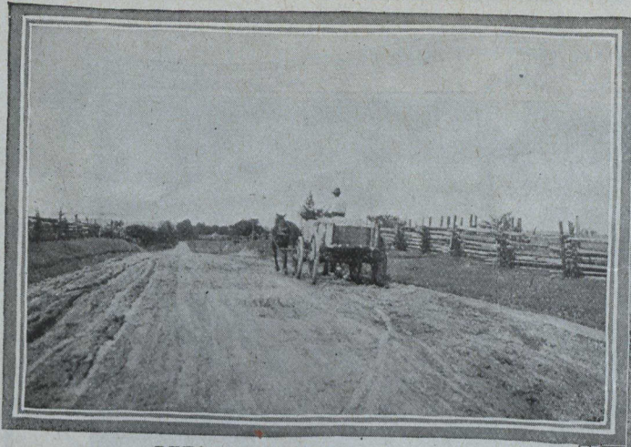
BEFORE USING TARVIA Queen Street, Newmarket, Ont. A slow, muddy highway into town.
