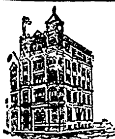
HEAD OFFICE BUILDING, MONTREAL
