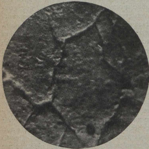
Fig. 1—White Lead Paint, Showing Chalked Condition
