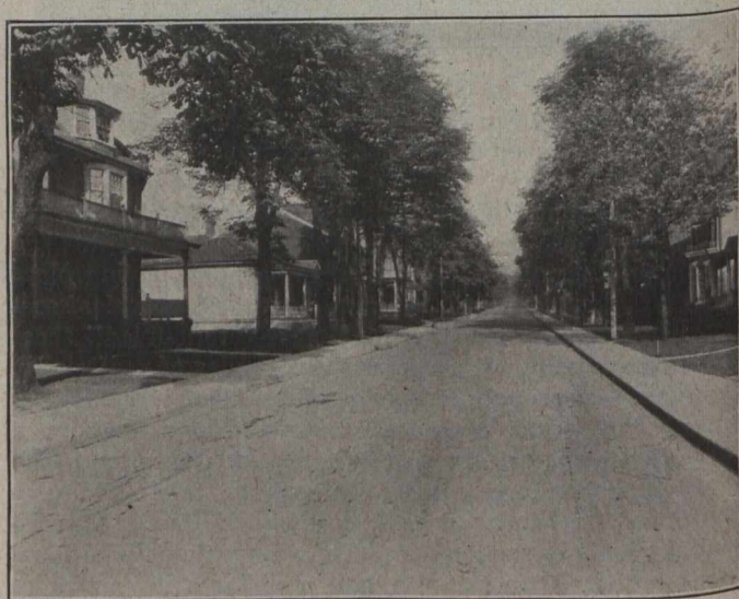
Seaton Street, Toronto, sheet asphalt, laid 1908, photo 1917. No repairs to date
