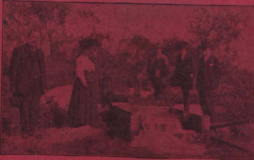
The illustration is of an Air Lift Pump, lifting 1361 gallons of water per minute, 31 feet, from a 12-inch well 270 feet deep.
