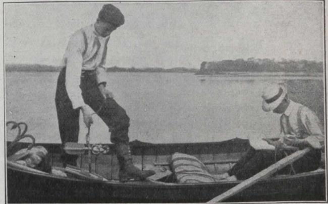
Metering with small Price current meter. The conical cups revolve fast or slow in response to the current, and revolutions are registered by an electric recorder, the time being taken by stop watch.
