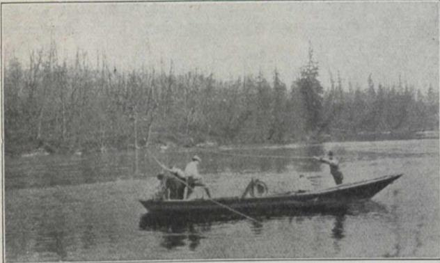
Metering with large Price current meter on the Montreal River, using cable for distance.
