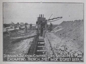
are saving large amounts for contractors al over Canada, United States and other countries. Every Parsons Excavator is equipped with extra large engines and boilers and the entire machine made of extra quality of steel, giving them the power and strength to handle any class of material or any size trench, without tearing or racking machine. The buckets are flexible, and self-cleaning of all material, with teeth that will cut anything except solid rock.
