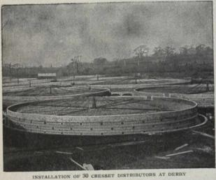
THE Sprinkler that holds its own in the home country because its frictionless air lock seal enables it to revolve with less head than any other. With a few inches head.
