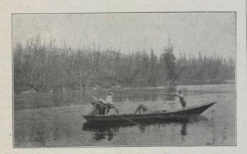
Metering with large Price current meter on the Montreal ... River, using cable for distance.
