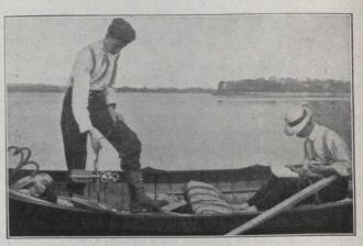
Metering with small Price current meter. The conical cups revolve fast or slow in response to the current, and revolutions are registered by an electric recorder, the time being taken by stop watch.
