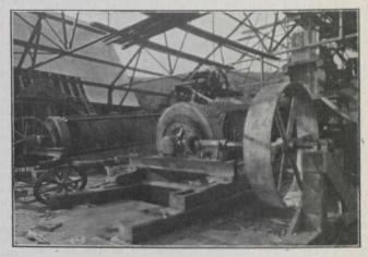
Screens 6 ft. x 22 ft. with 2½ in. openings (during construction).
