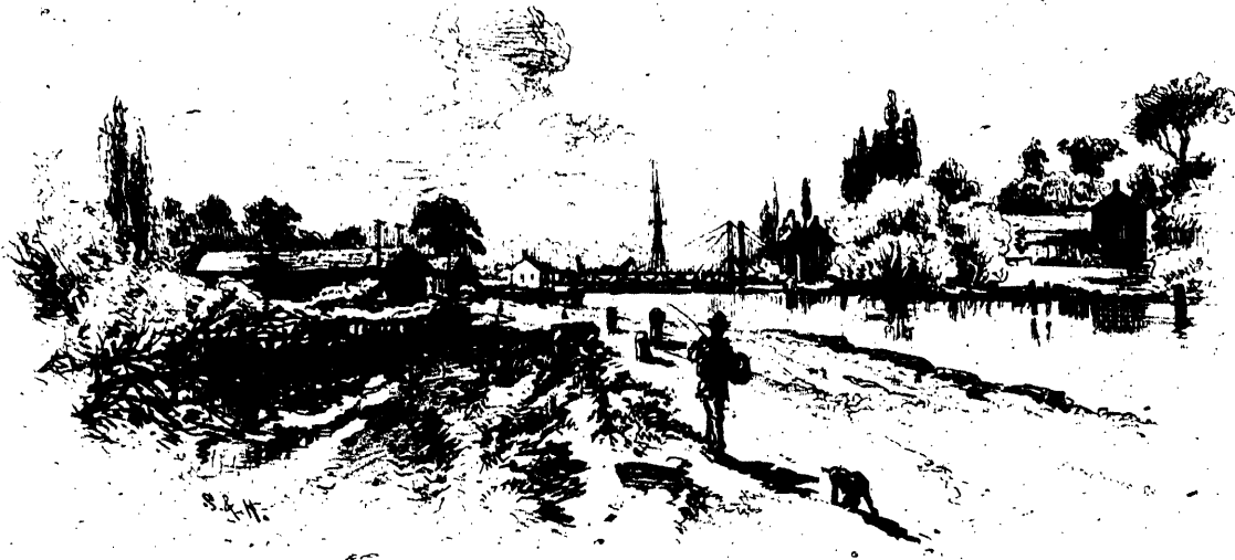
NEAR LOCK No. 2 OLD CANAL.
