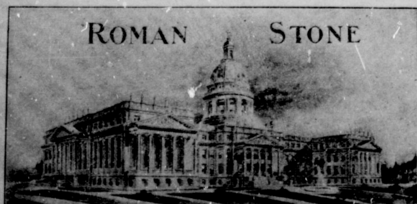
NEW ARTS BUILDING, UNIVERSITY OF OTTAWA Roman Stone was Specified in this Building
