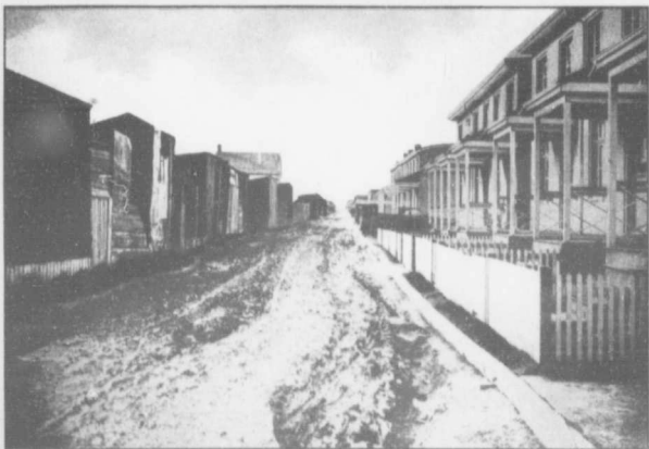
Row of houses for artisans, located in a "lane" facing outbuildings as shown on left.
