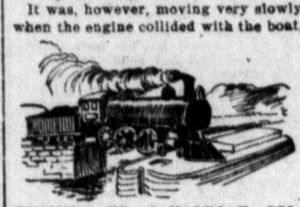
ENGINE AND CANALBOAT COLLIDED.
