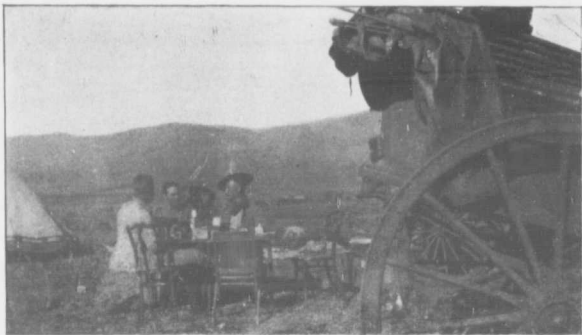
D BATTERY MESS.
