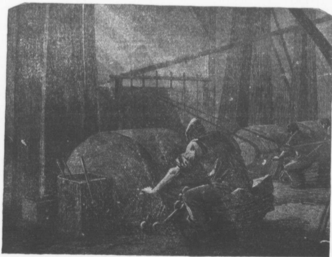
GRINDING THE GUN-BARRELS.
