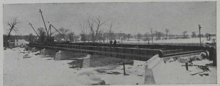
View of Abutments, Piers and Superstructure Partly Completed.
