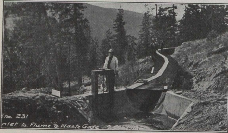
Inlet to Flume and Waste Gate.
