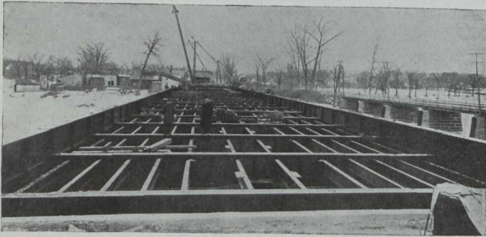
View of Bridge Under Construction, Showing Floor Beams and Stringers.
