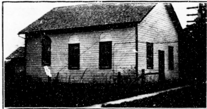
Head Office Burgessville Telephone Co.
