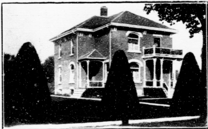
Residence of Mr. M. Bushell.
