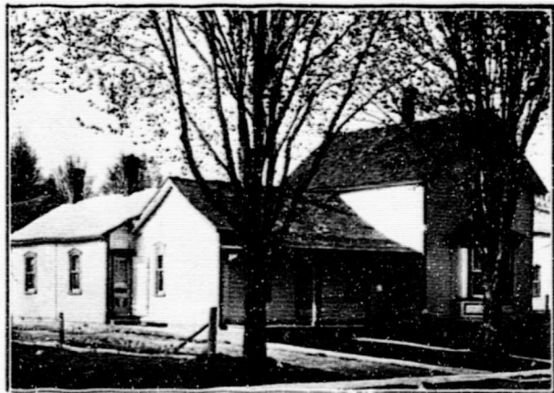
Residence of Mr. Arden Cameron.
