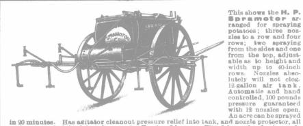
This shows the H. P. Spramotor arranged for spraying potatoes; three nozzles to a row and four rows; two spraying from the sides and one from the top, adjustwidth up to 40-inch rows. Nozzles absolutely will not clog. 12 gallon air tank. Automatic and hand controlled, 100 pounds
