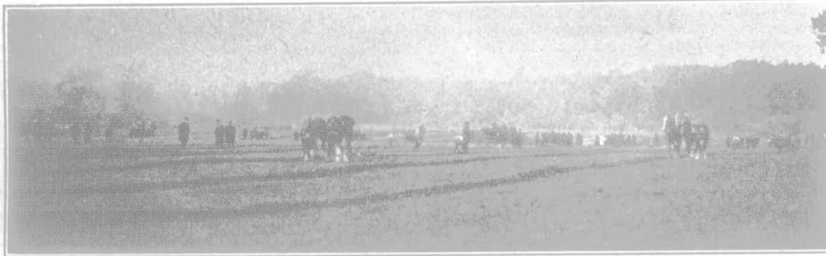
Men with High-cutting Plows Getting Started.
