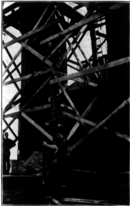
Bettington Boilers of Waterford Lake power-house, in course of construction.
