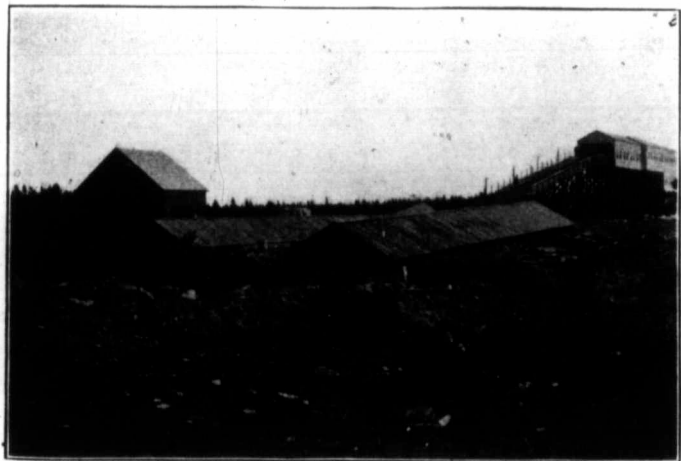
Completed Bankhead and slopes of modern Colliery No. 14.
