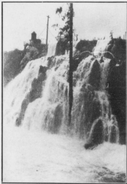
Stave Lake Falls, showing source of Western Canada Power Company's supply of electrical energy.
