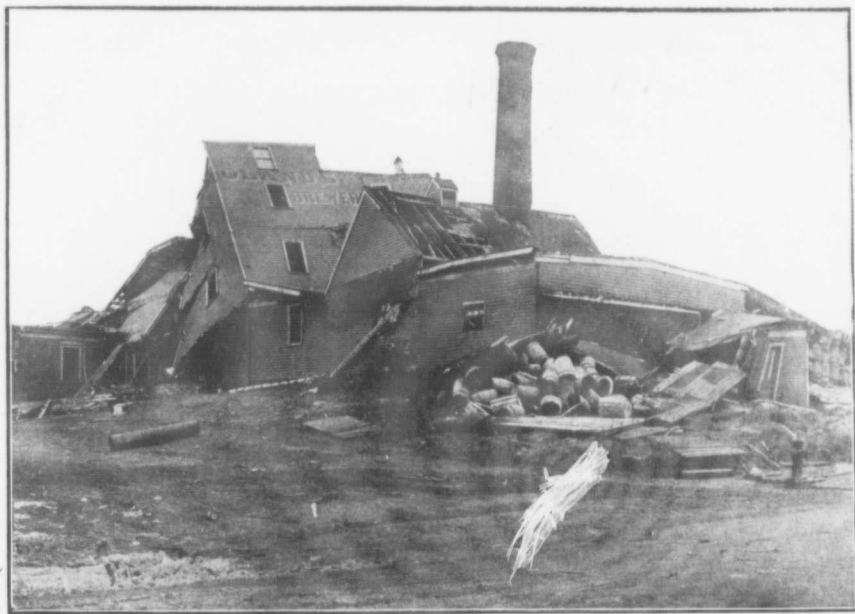
Oland's Brewery. This building is a complete wreck and all that remains standing is the smoke stack.
