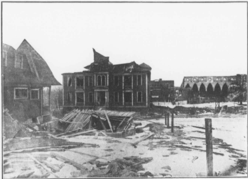
A view of the wrecked St. Joseph's School, with the ruins of St. Joseph's Church showing in the rear.
