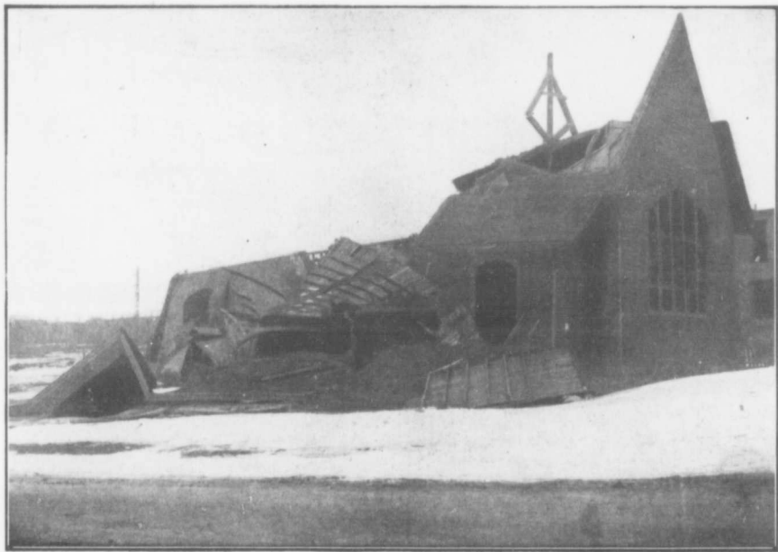
The ruins of Emmanuel Episcopal Church, Dartmouth. As will be seen by the picture this building is a complete wreck.
