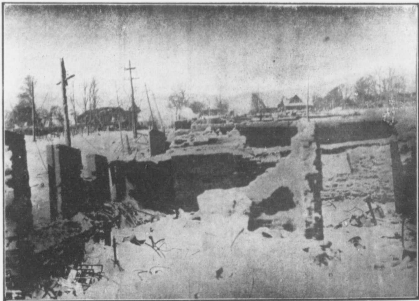
This is a scene at Richmond which shows how completely the buildings in that section were demolished.
