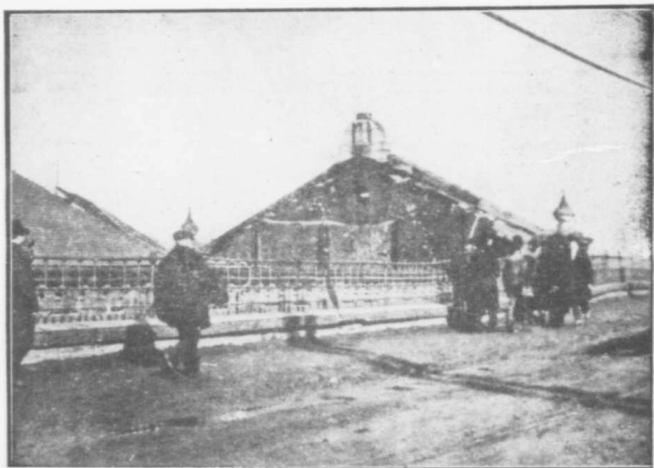
This view is looking down on the roof of North Street Station and shows how that building was battered up.
