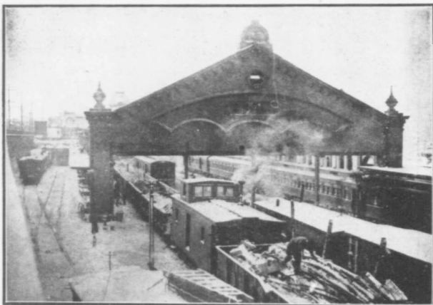
This is the interior view of North Street Station after the explosion, showing the roof smashed in and wreckage trains carrying debris away.
