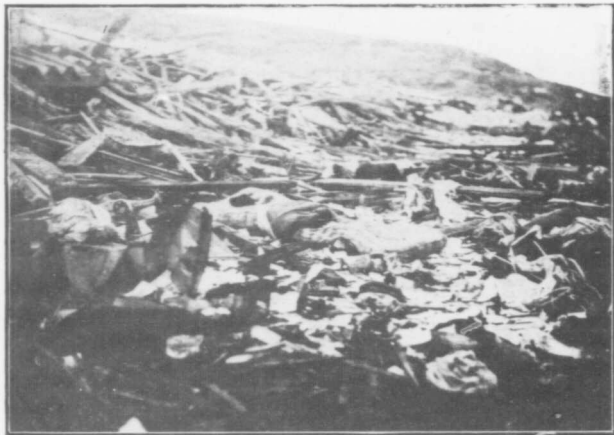
Wreckage of homes in the devastated area.
