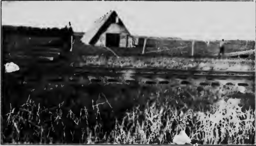
(a) Triangular shed for storage of dried peat, government peat bog, Alfred.
