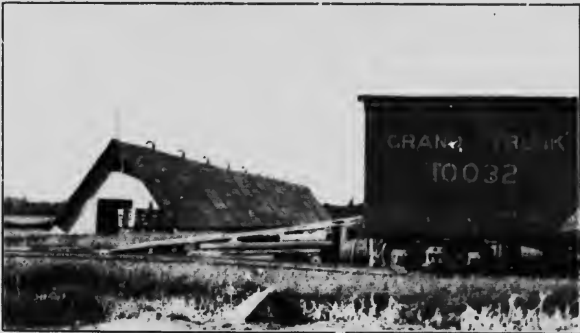
(b) Siding and platform for loading of peat into railway cars, government peat bog, Alfred.
