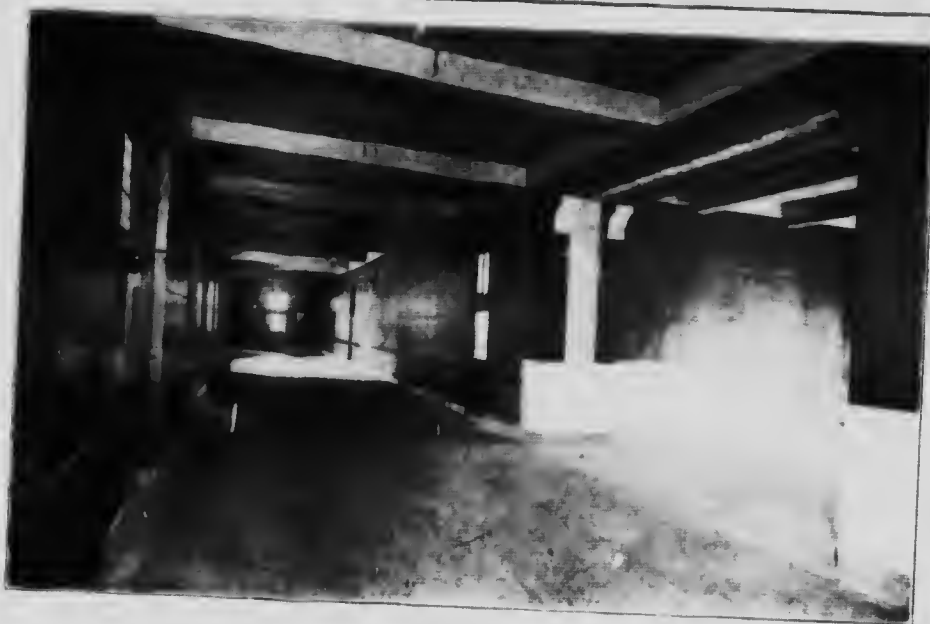
FIG. 6. CORRIDOR, LAVALLETTE SCHOOL W. B. HIND, Architect
