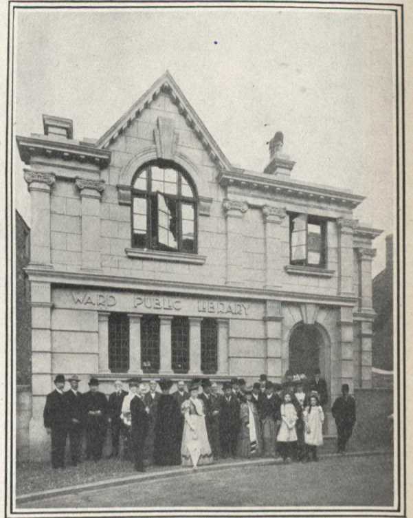
The Public Library at Peel, Isle of Man, erected by Mr. J. K. Ward, of Montreal.
