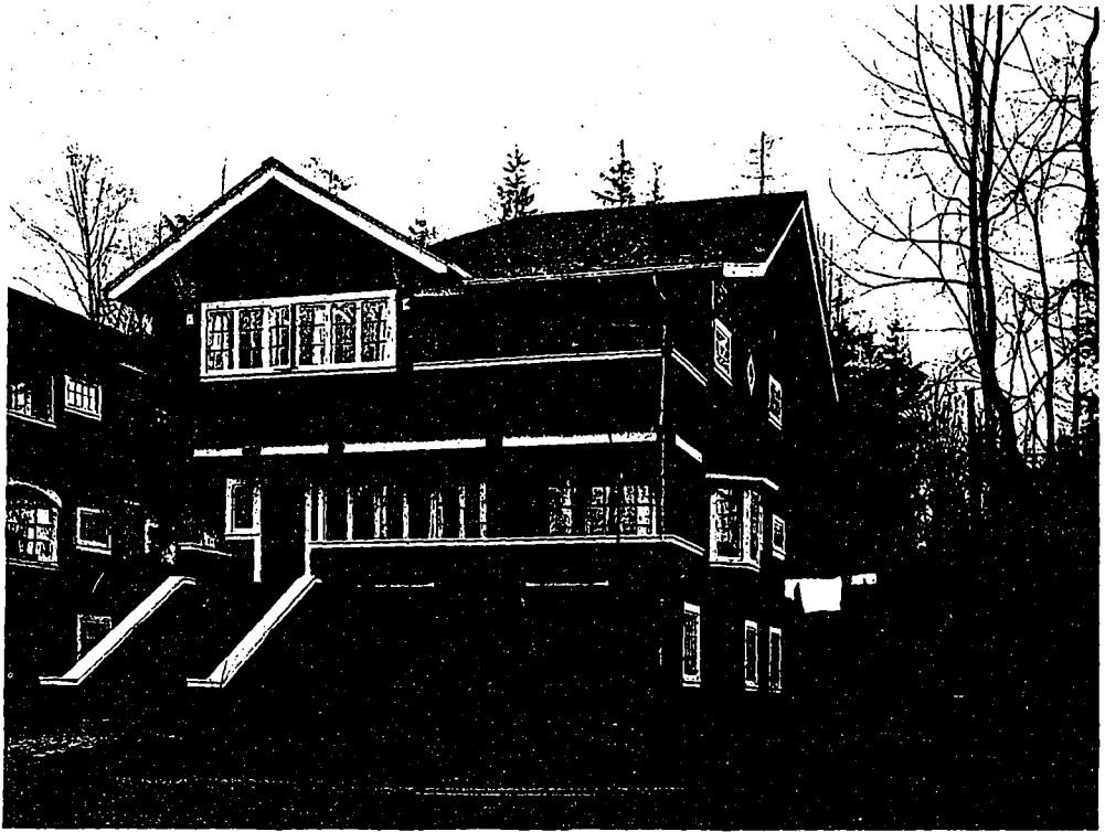
Residence of W. O. Webster, Vancouver, B.C.—While Characteristic of the Bungalow in Design, this House is Placed on a High Foundation, in Order to Take Full Advantage of the View Which its Site Commands. E. Stanley Mitton, Architect.
