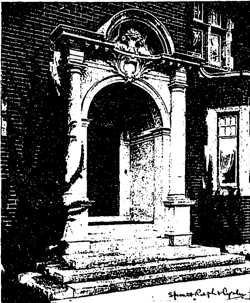
Detail of Entrance, Residence of Mr. E. R. Wood, Toronto. Sproatt & Rolph, Architects.
