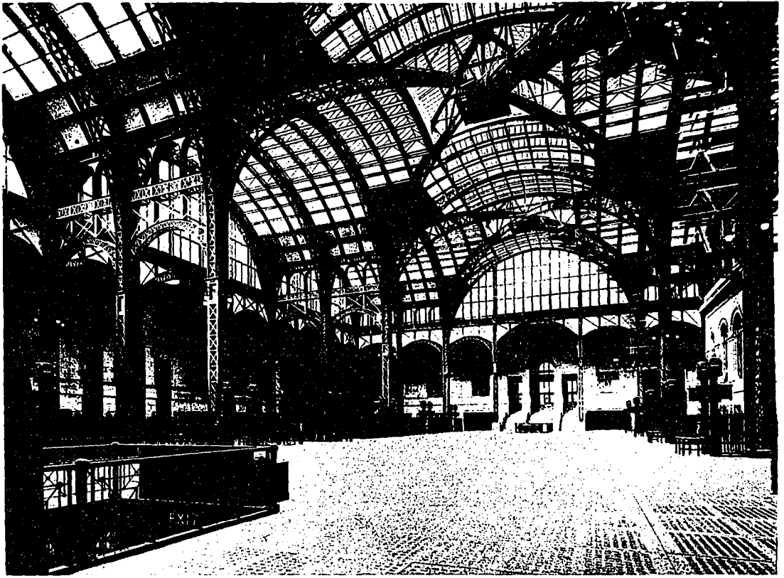
Upper Portion of Concourse, Pennsylvania Terminal, Showing the Steel Framework and Overhead Glass Enclosure. McKim, Mead and White, Architects.
