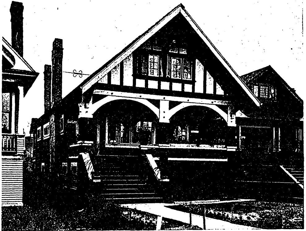
Bungalow of H. J. Simmons, Vancouver, B.C.—The Low, Broad Lines and Massiveness of the Design, make the Heavy Timber Effect and External Construction of this Dwelling Eminently Suitable. E. Stanley Mitton, Architect.
