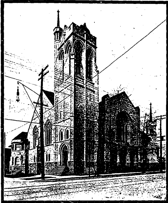
A Sand-Lime Ecclesiastical Edifice—High Park Presbyterian Church, Roncesvalles Avenue, Toronto. Smith and Gemmell, Architects.
