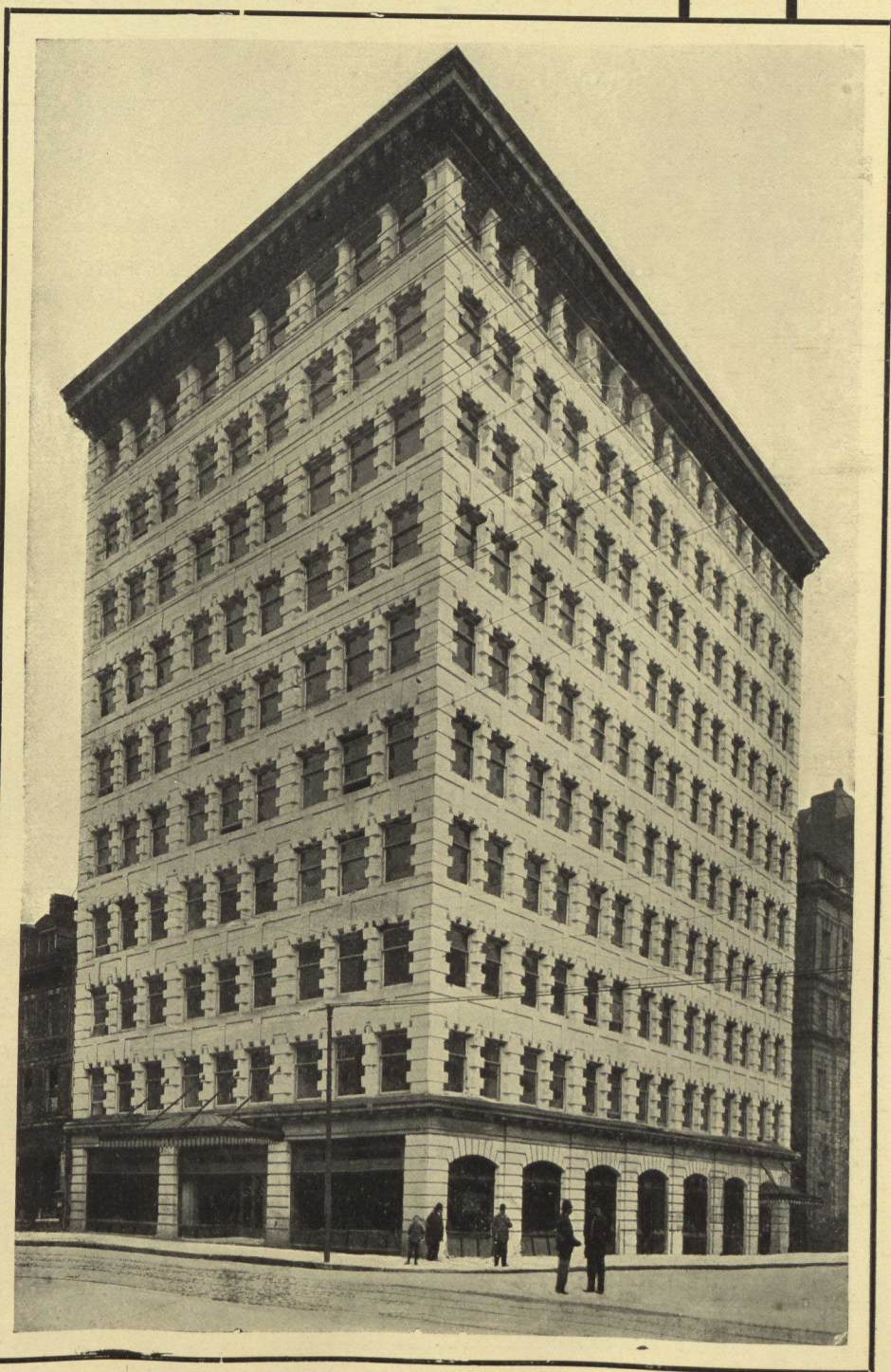
The Lumsden Building, Yonge Street, Toronto. J. A. MacKenzie, Architect. This building was FIRE-PROOFED throughout with DON VALLEY POROUS TERRA COTTA.
