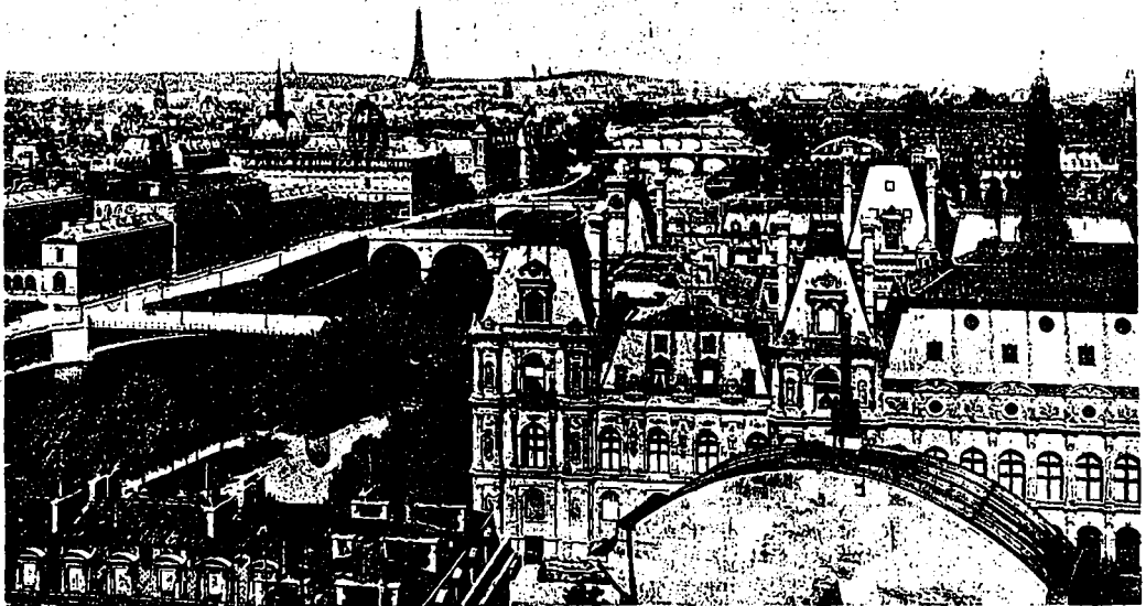
General View, Looking Down the Seine—Showing the Frequency With Which Bridges Occur.
