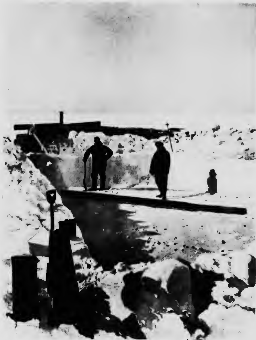
DIGGING THE FOUNDATIONS OF FRAMHEIM.
