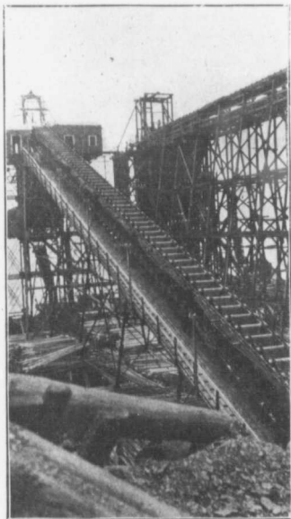
LOADING PIER SHOWING CONVEYORS, WABANA.
