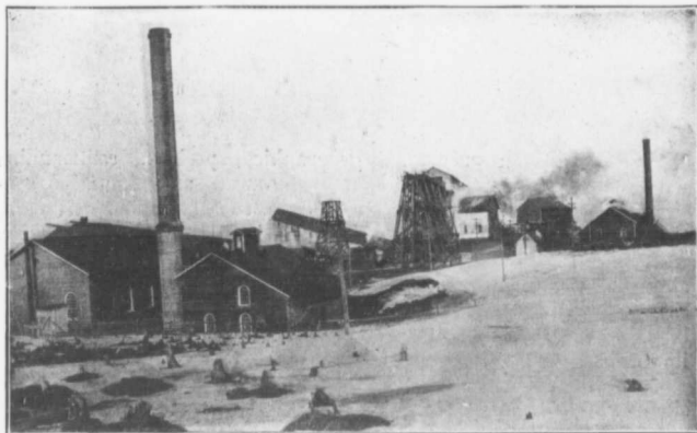
ENGINE HOUSE AND DECKHEAD, SUBMARINE MINE, WABANA.
