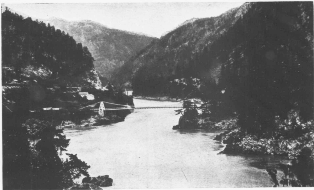
CARIBOO BRIDGE, FRASER RIVER
