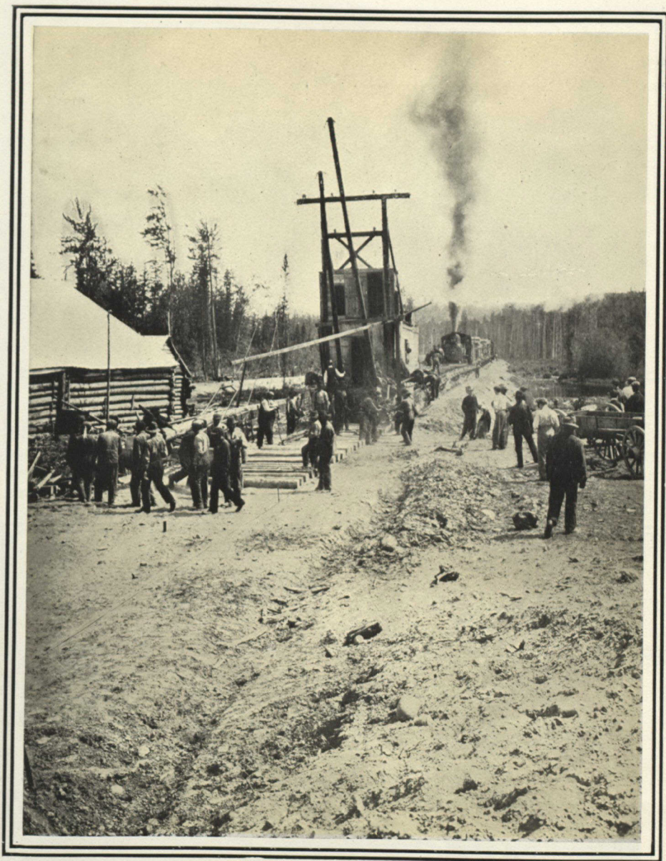
THE ADVANCE GUARD OF THE TRACK LAYERS
