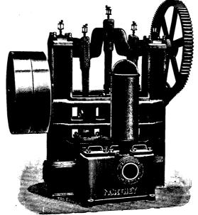
We illustrate in this advertisement a typical Pump for Mine Work. This is our Triplex Power Pump, fitted with tight and loose pulleys as shown in cut. It is the regular Triplex type with the three cranks 120 degrees apart; crankshaft and connecting rods are of steel; gears machine-cut from the solid; plungers of brass and ail details carefully worked out. This Pump is especially adapted for service with Electricity as the motor power.
