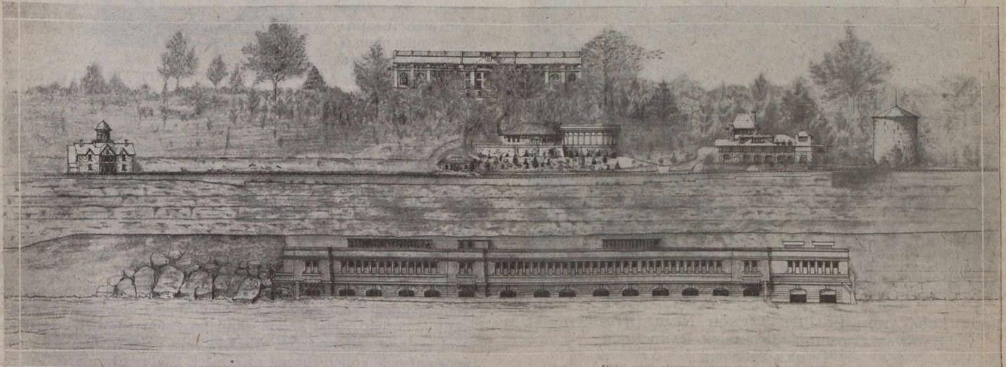
ELEVATION SHOWING POWER HOUSE AT FOOT OF CLIFF—EXTENSION AT THE RIGHT—ON BANK, FROM LEFT TO RIGHT, TABLE ROCK HOUSE, NO. 1 AND NO. 2 SURGE TANKS, REFECTIONARY, AND NEW SURGE TANK AT EXTREME RIGHT—ABOVE, DISTRIBUTING STATION
