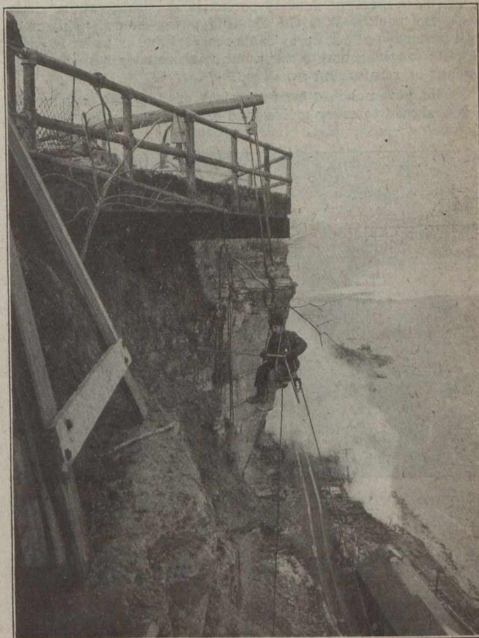
SCALING LOOSE MATERIAL FROM CLIFF ABOVE POWER HOUSE SITE—INTERNATIONAL ARCH BRIDGE IN DISTANCE
