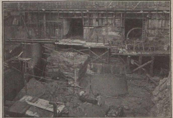
POWER HOUSE EXTENSION SITE READY FOR FORMS—TWO TUNNEL PORTALS APPEAR IN BACKGROUND, WITH PEN-STOCK NO. 16 BEING ASSEMBLED—DRAFT TUBE FORM FOR NO. 15 IN POSITION AT LEFT
