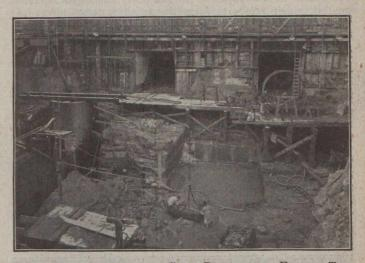
POWER HOUSE EXTENSION SITE READY FOR FORMS-TWO TUNNEL PORTALS APPEAR IN BACKGROUND, WITH PEN-STOCK NO. 16 BEING ASSEMBLED-DRAFT TUBE FORM FOR NO. 15 IN POSITION AT LEFT
