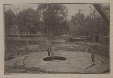
SURGE TANK FLOOR ASSEMBLED READY TO LOWER ONTO FOUNDATION
