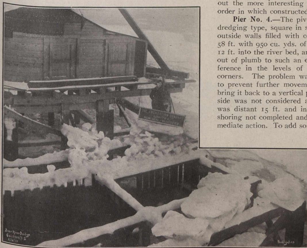
Fig. 1.—An Illustration of Ice Conditions During the Sinking of Caisson No. 5.
