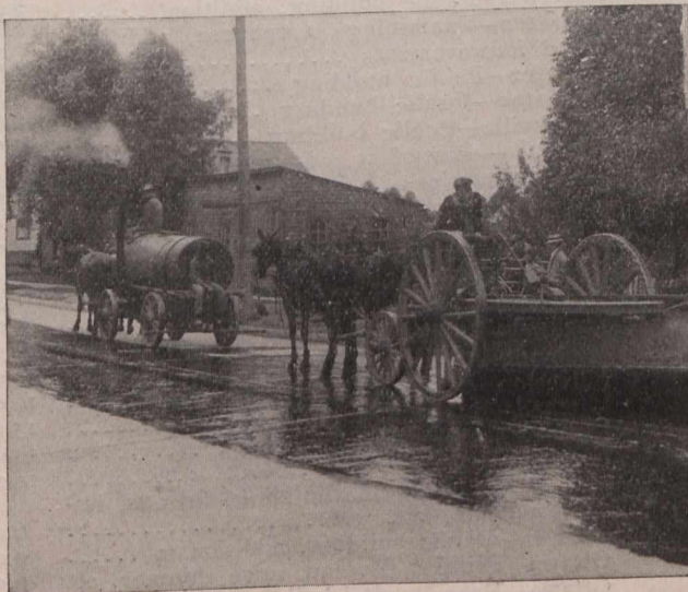
One of the methods of applying and spreading Dolarway Bitumen on Concrete Base.
