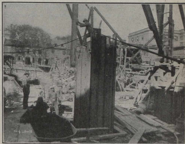
Driving Steel Sheeting, General Hospital, Montreal.
