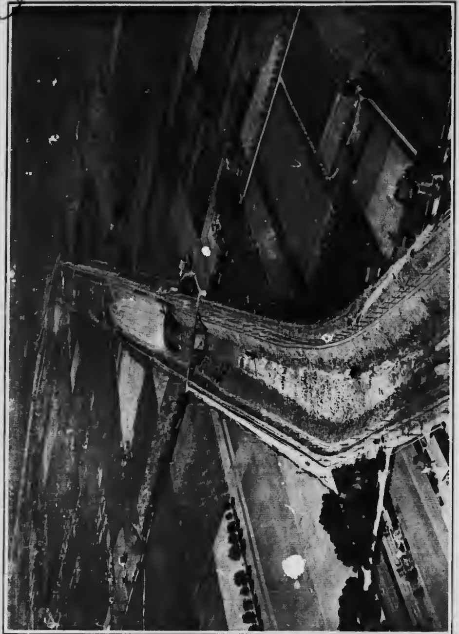
Aeroplane view of the Power Canal, Chippewa-Queenston Power Development.
