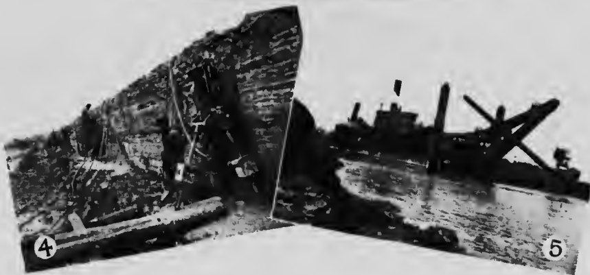
(1) Cableway Excavator in Welland River. (2) Cableway excavator from East Bank of Welland River. (3) Site of the World's Largest Power House. (4) Drilling wall of Forebay. (5) Dredge loading a scow opposite Hog Island, at the mouth of the Welland River.
