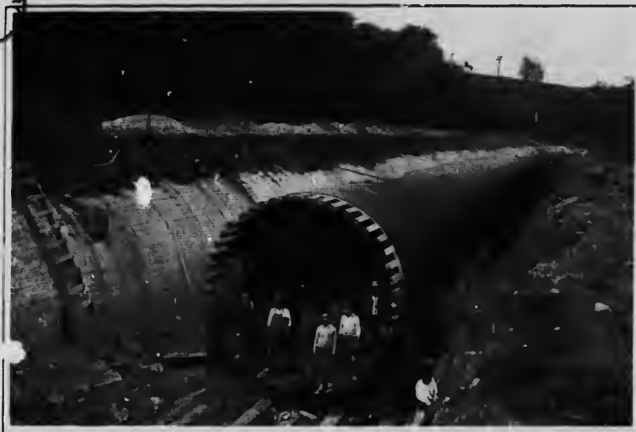
Wood Stave Pipe Line during Construction.
