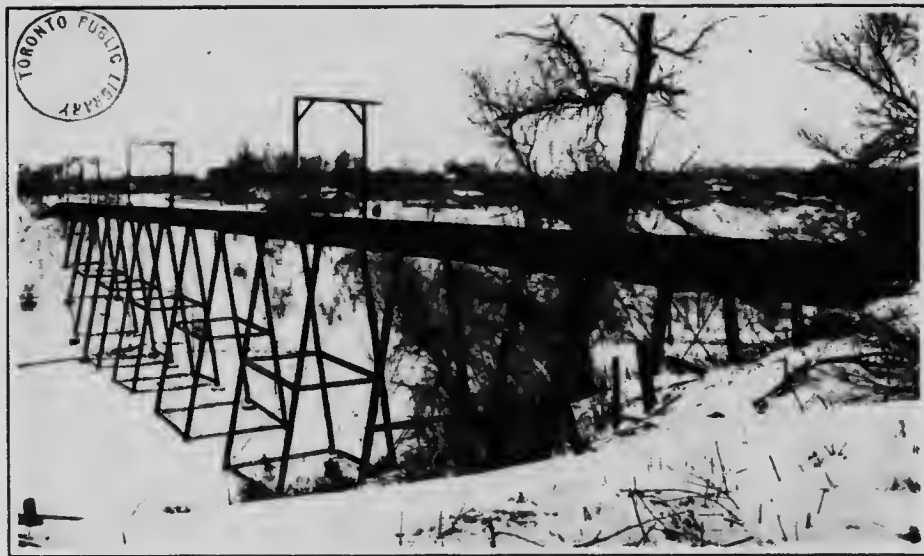
A Steel Trestle on the London and Port Stanley Railway.
